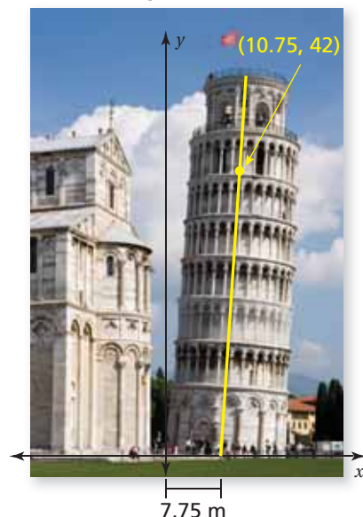
Leaning Tower of Pisa
